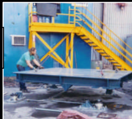
Installing a coil scale
